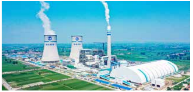
Yicheng Power Plant
