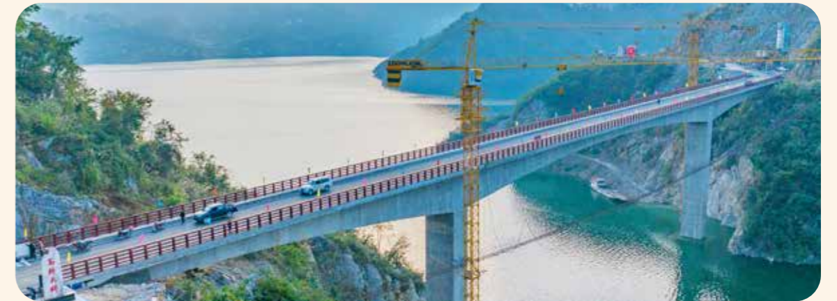
Gaoqiao Bridge completed and open to traffic
