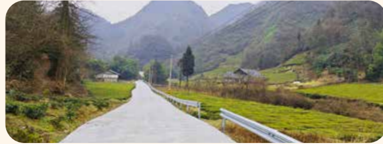
Repaired road of Beizhen Village
