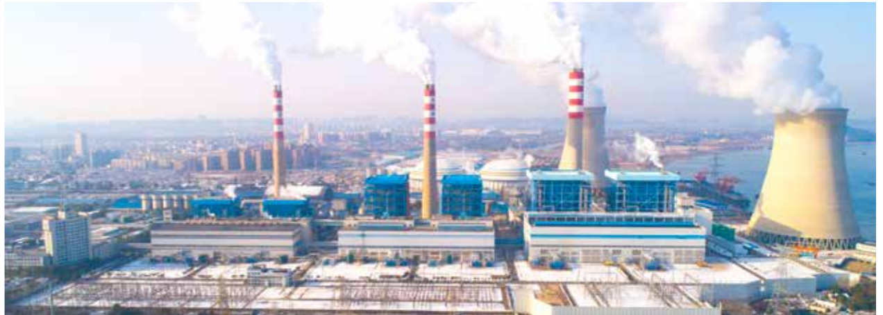
Ezhou Power Plant
